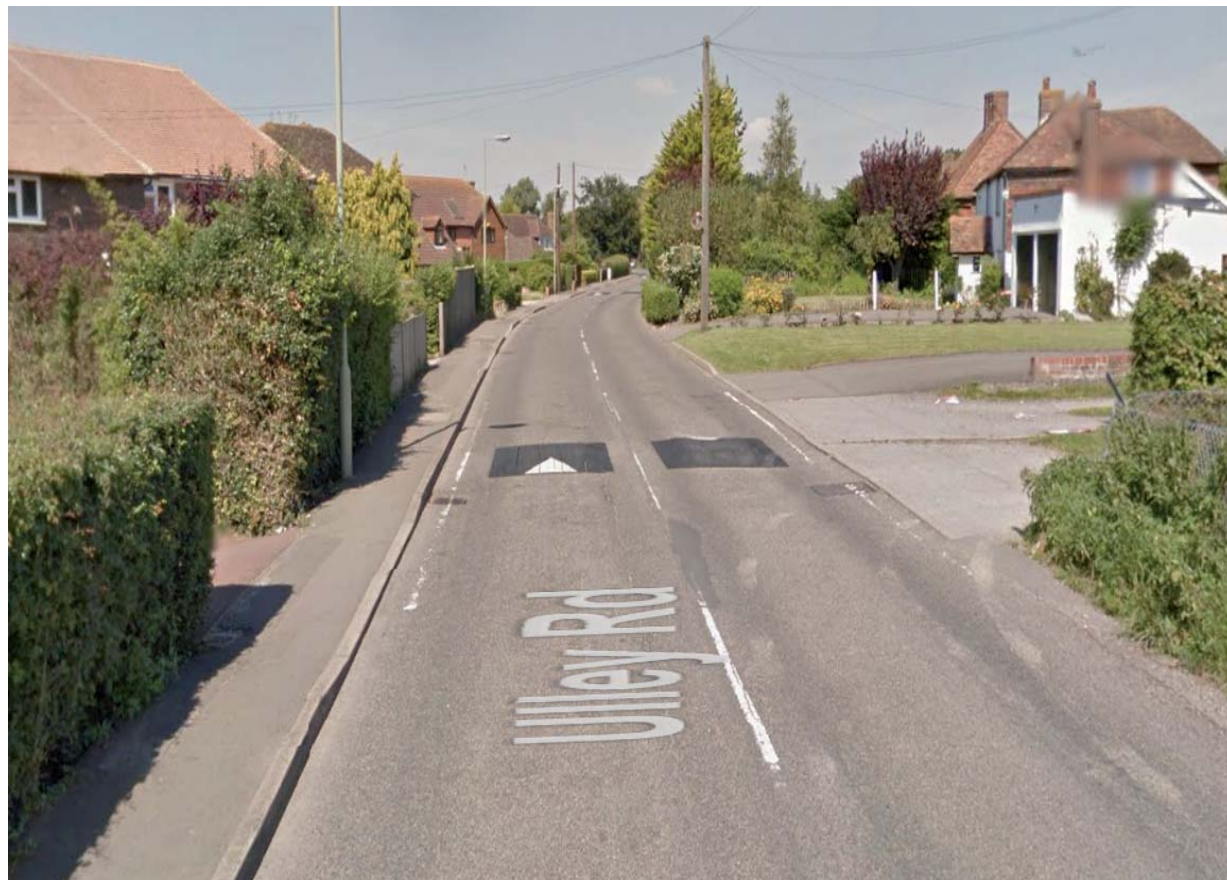
Below: View looking north west along Ulley Road, Kennington with speed bumps installed
