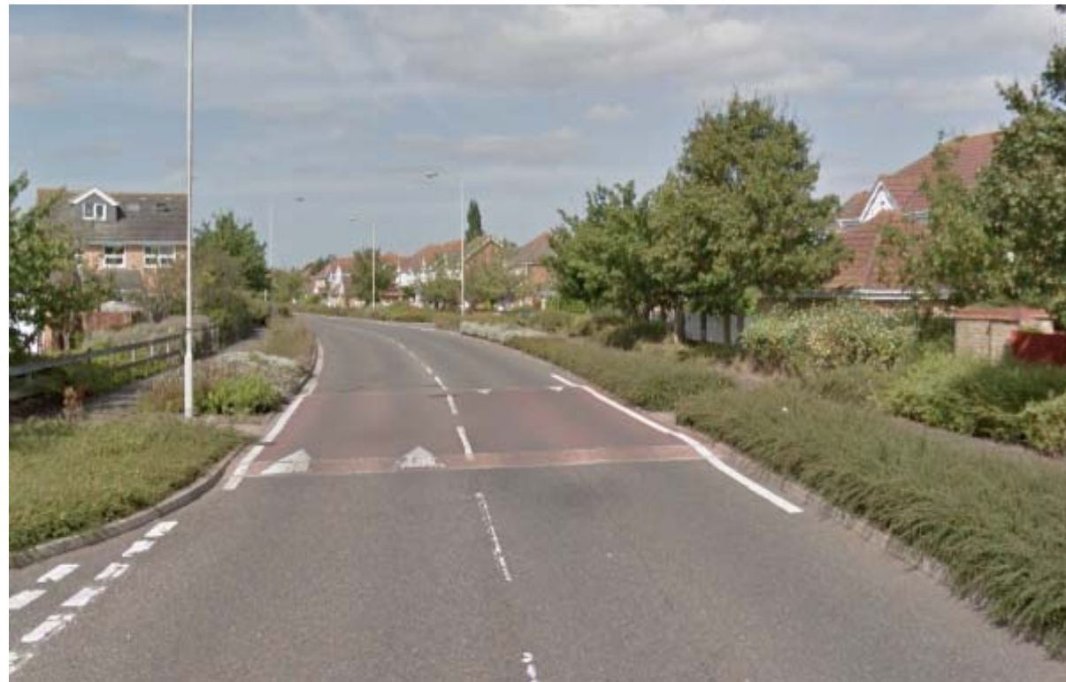
Above: View looking north west along Roman Way, Park Farm to illustrate alternative speed bump design
